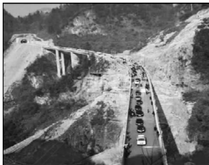
FIGURE 21 - THE BRIDGE WITH CONDUCTIVE CONCRETE DEICING TECHNOLOGY
