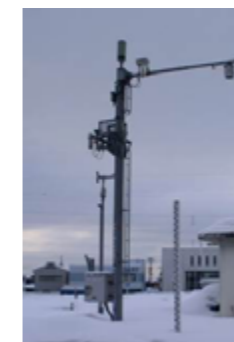
ROAD WEATHER STATION
