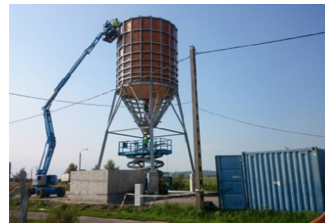
SALT STORAGE SILO; HUNGARIAN PUBLIC ROAD NON-PROFIT PLC
