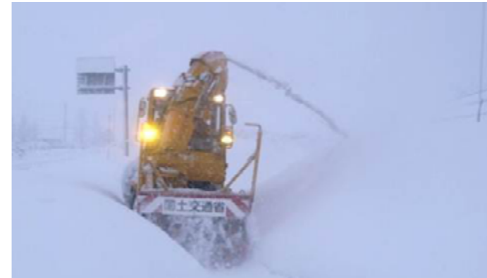
FIGURE 6 - SIDEWALK SNOW REMOVAL
