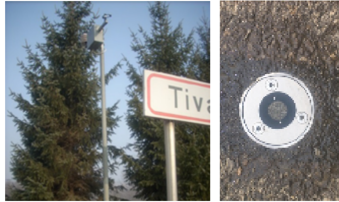
WEATHER SENSOR, TELECOMMUNICATION COMPONENT AND ROAD PAVEMENT SENSOR BELONGING TO THE ÚTMET ROAD AND WEATHER INFORMATION SYSTEM'S STATION; HUNGARIAN PUBLIC ROAD NON-PROFIT PLC
