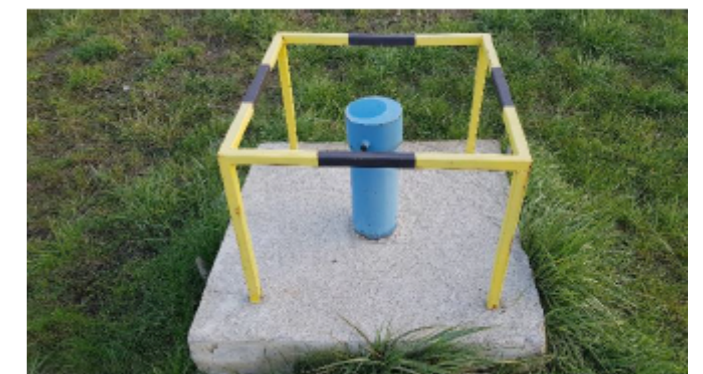
GROUNDWATER MONITORING WELLS; HUNGARIAN PUBLIC ROAD NON-PROFIT PLC
