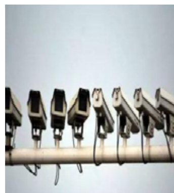
ROAD SURVEILLANCE CAMERA
