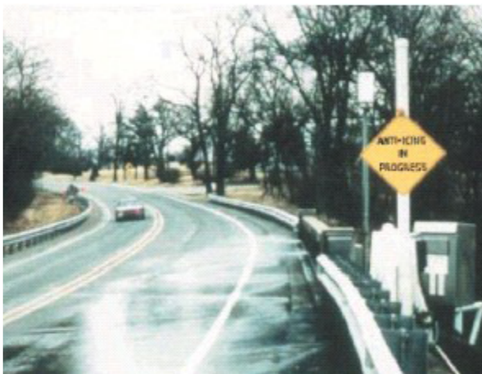
FIXED ANTI-ICING SPRAY SYSTEM (PHOTO COURTESY OF CRYOTECH DEICING)
