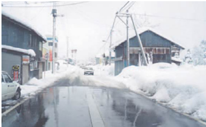
FIGURE 11 - EFFECT OF SNOW-MELTING SPRINKLER SNOW-FLOWING GUTTER
