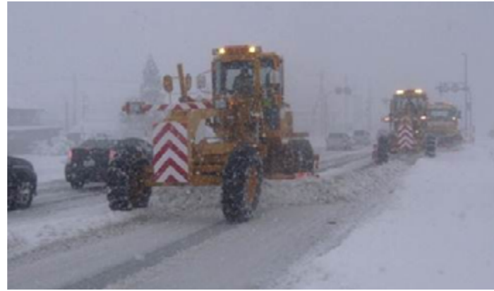
FIGURE 5 - MULTI-LANE SNOW REMOVAL
