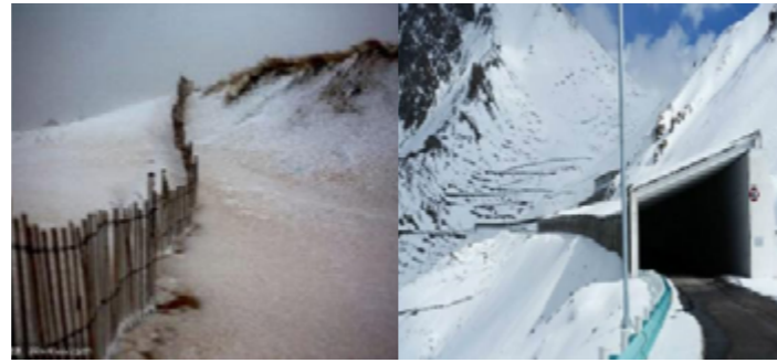
SNOW FENCE SNOW SHED FIGURE 15 – SNOW CONTROL MEASURES
