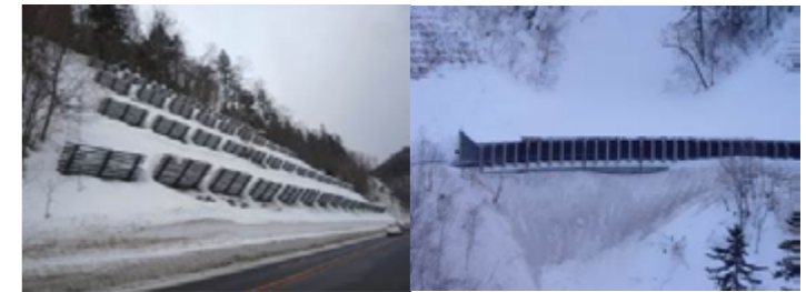
AVALANCHE CONTROL FENCE
