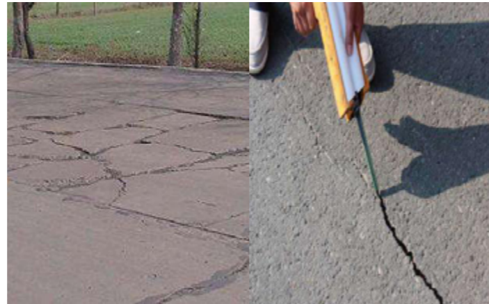
FIGURE 12 - ROAD CRACKS REPAIRING
