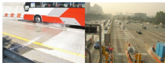
AUTOMATIC SPRINKLING SYSTEM(BRINE)
