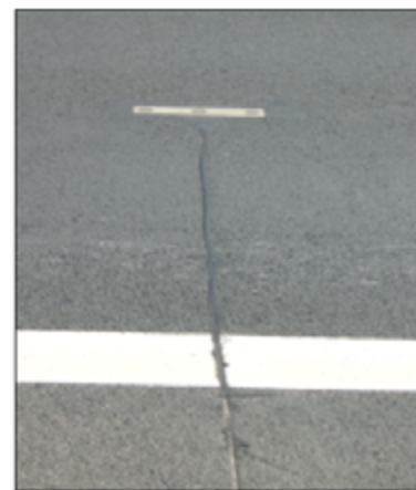
road surface sensors
