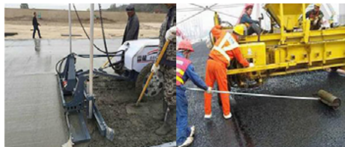
FIGURE 11 - GROUND LEVELING AND CONSTRUCTIONS OF SURFACE
