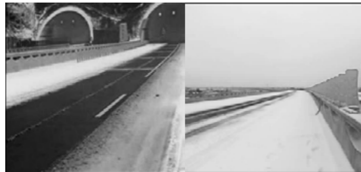
FIGURE 22 - THE BRIDGE DECK WITH (LEFT) AND WITHOUT ANTI-ICING MATERIAL (RIGHT)
