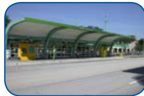
Extended bus platform on Miami-Dade Transitway
