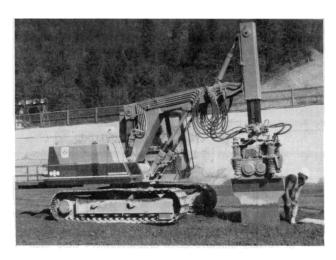
Figure 9-4. Contract joint placement using a vibrating blade to insert galvanized steel sheeting
