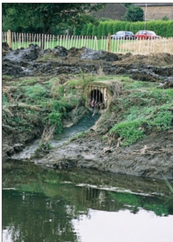
Typical outfall before replacement
