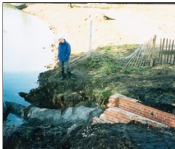
New outfall chamber under construction
