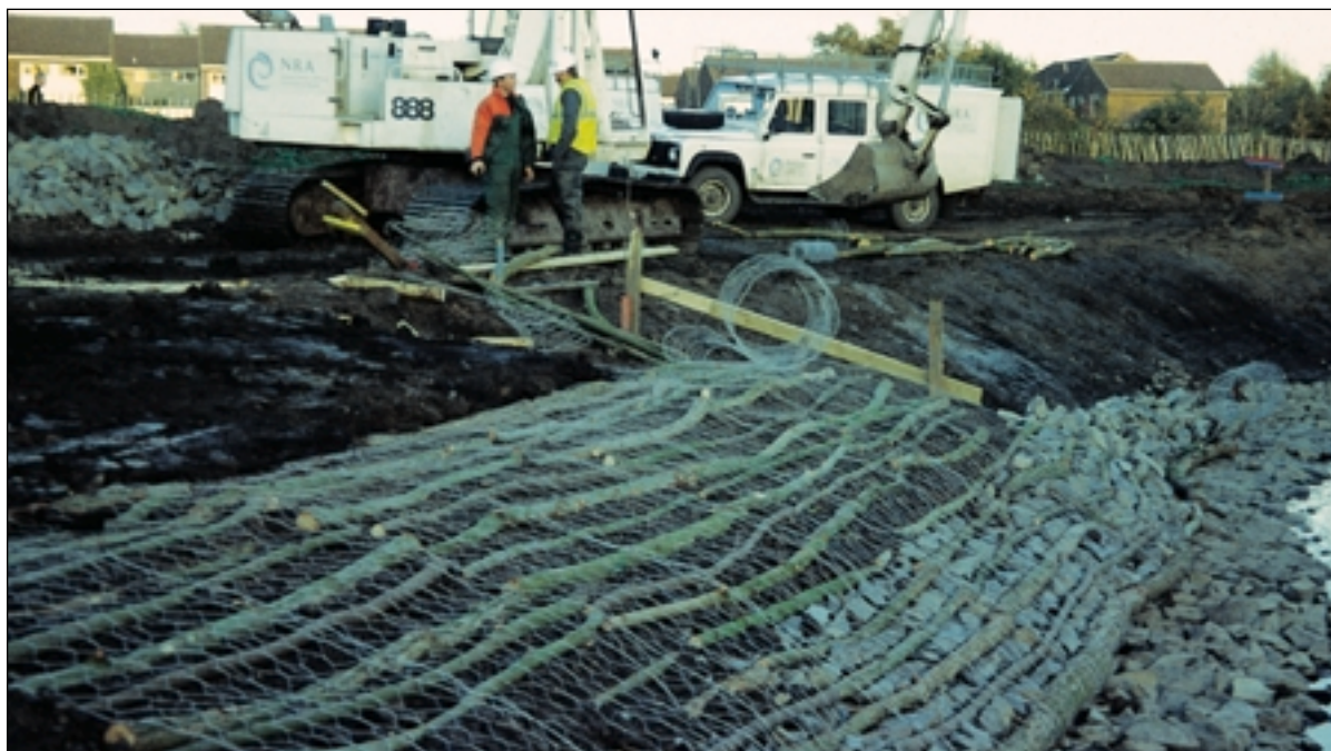
Mattress revetment under construction – October 1995
