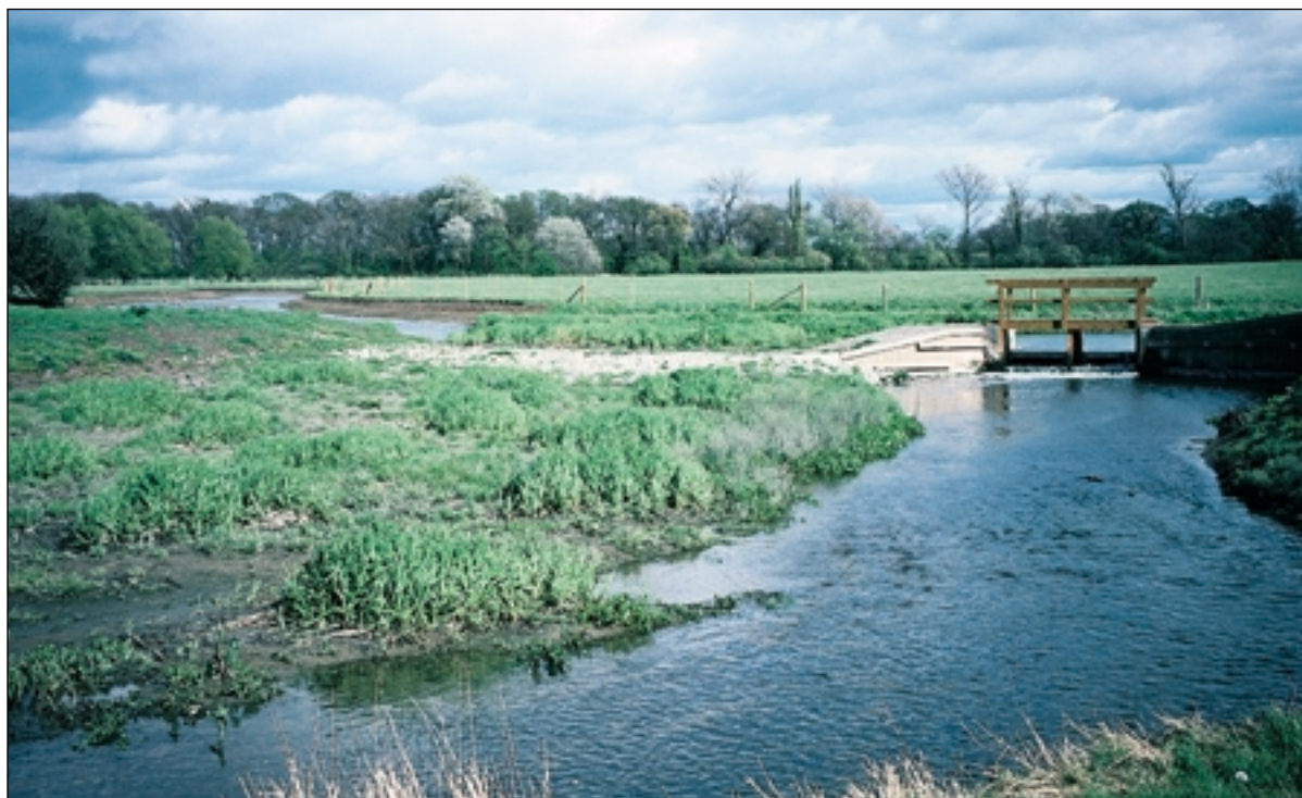
Spillway alongside bifurcation weir – April 1997
