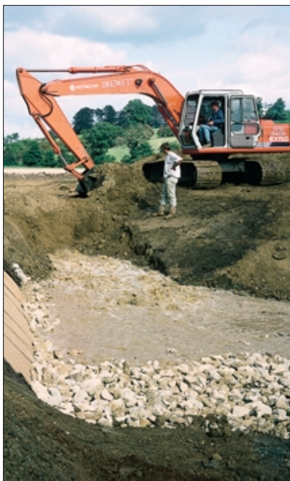
Construction of coir matting revetment – river being released
