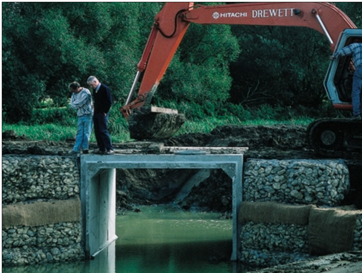
New concrete culvert crossing under construction
