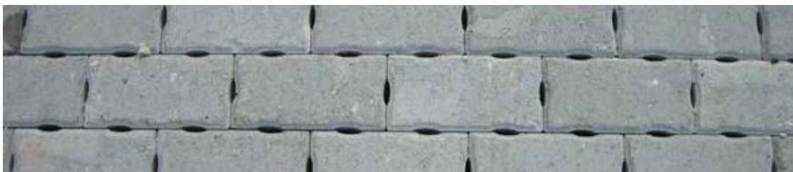
Figure 8. Selected concrete block geometry.
