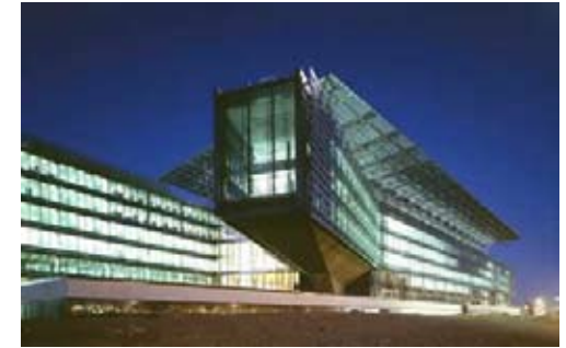
Endesa Headquarters Madrid, Spain 2004
