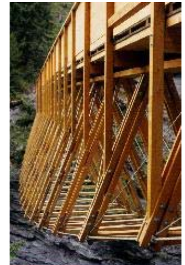
Transversiner Bridge Viamala, Switzerland, 1996
