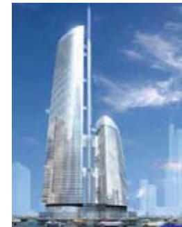
Federation Building Moscow, Russia, under construction
