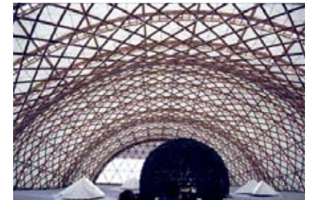
Japanese Pavilion at the Expo 2000 Hanover, Germany, 2000
