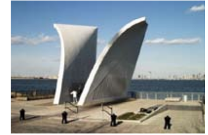
Staten Island September 11th Memorial Staten Island, New York 2004
