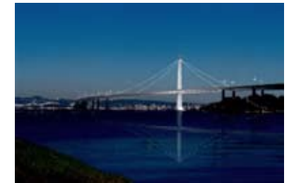
San Francisco- Oakland Bay Bridge San Francisco, California 2008
