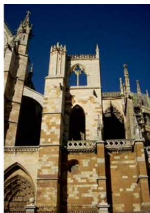
(a) Vista exterior
