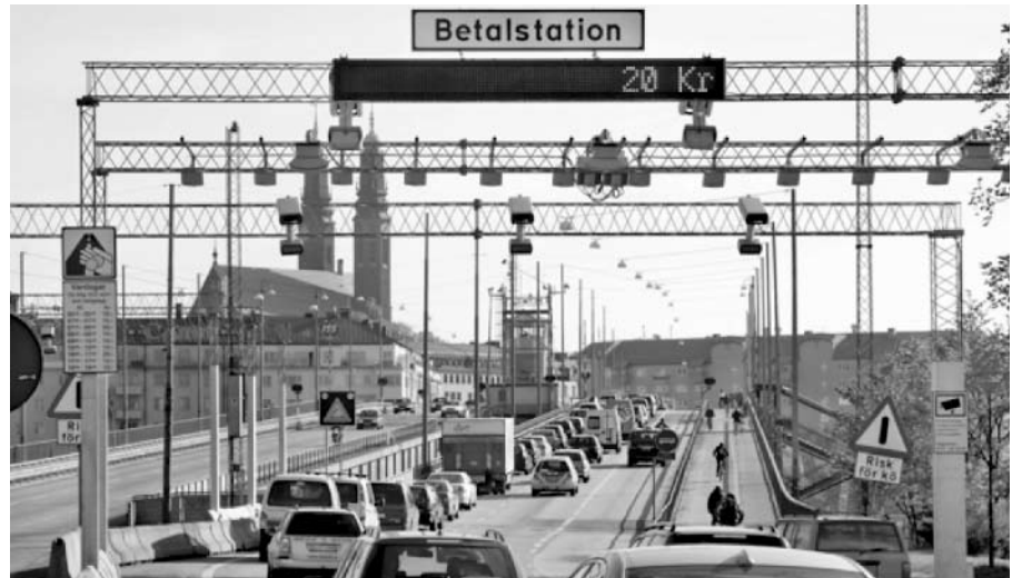
Figure 7. One of 18 control points using the three-gantry electronic toll collection system.
