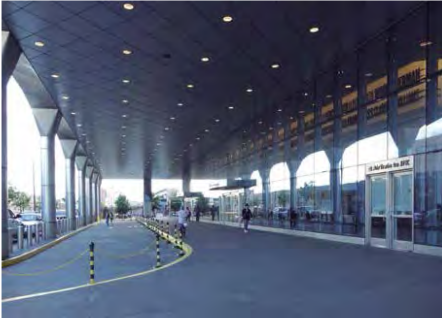
Fig. 1. Jamaica Station, Nueva York, Air Train a JFK Airport
