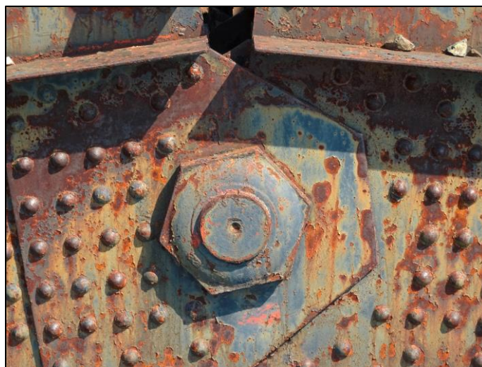
Figure 4.1.3.6 Close up Photograph of Arcola Bridge Pin Detail.
