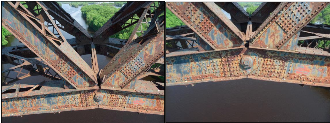
Figure 4.1.3.4 Photograph of Arcola Bridge Pin Detail. Figure 4.1.3.5 Photograph of Arcola Bridge Pin Detail
