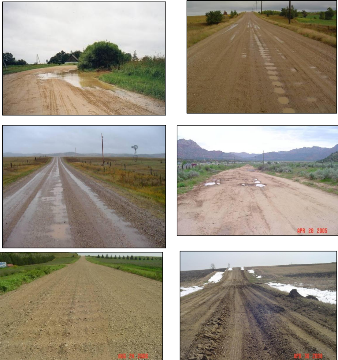
Figure 4.1.5.1. Unpaved roads and road condition. The images of top row show two roads in good condition. The roads shown in the images of the two middle rows demonstrate significant surface distresses, such as potholes, loss of crown, resulting water trapped on surface after rainfall which in turn further deteriorating roads in they are not properly repaired. The last row gives examples of roads with corrugation effects and severe rutting.
