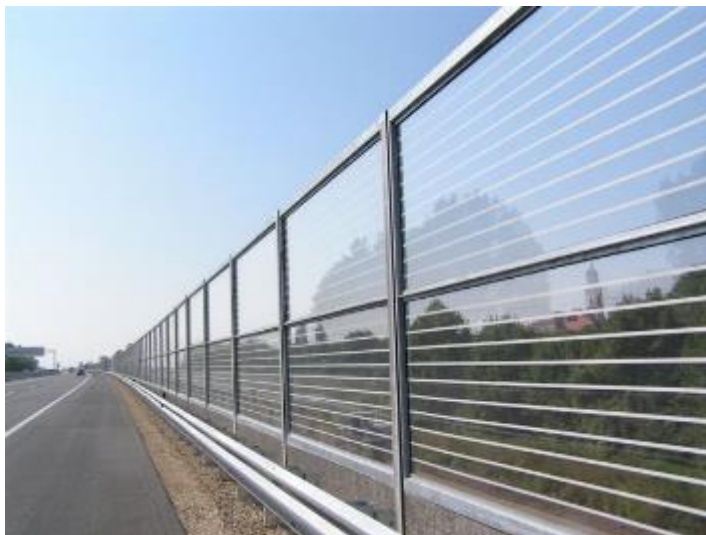
Figure 73: Example of a transparent noise barrier. A31 Valdastico, Vicenza, Italy.
