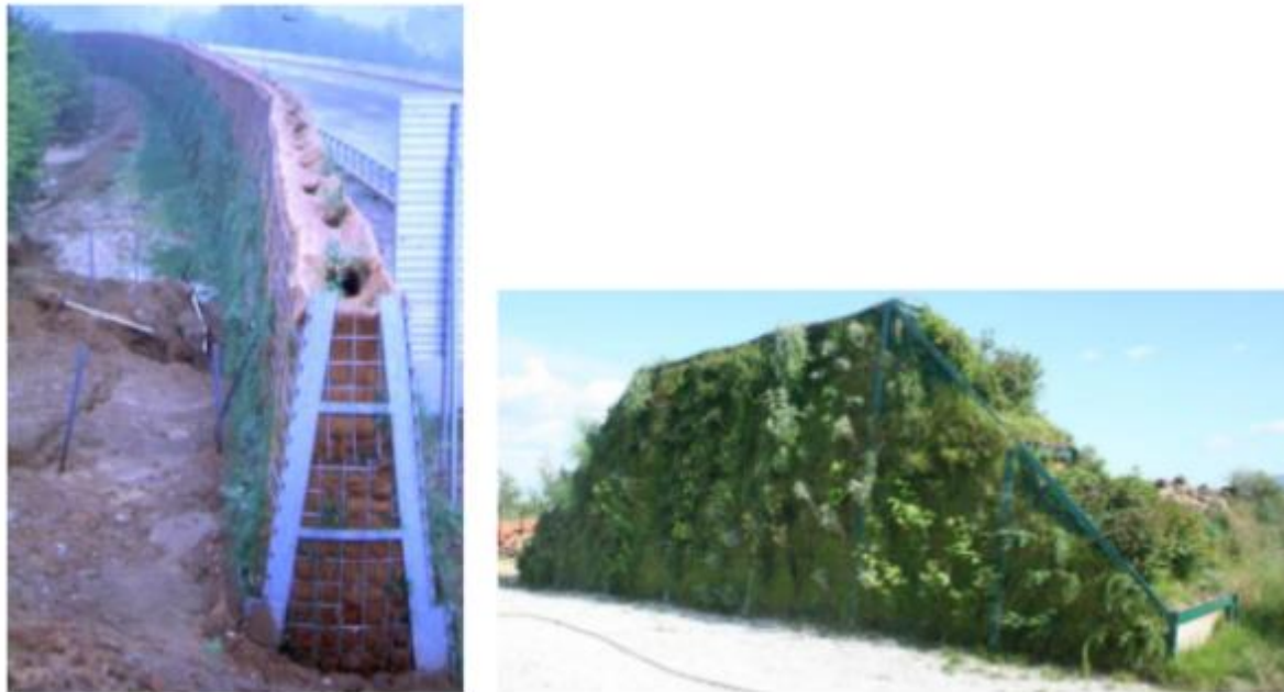
Figure 85: Bio barrier with metal structure (after construction and fully vegetated). [165]
