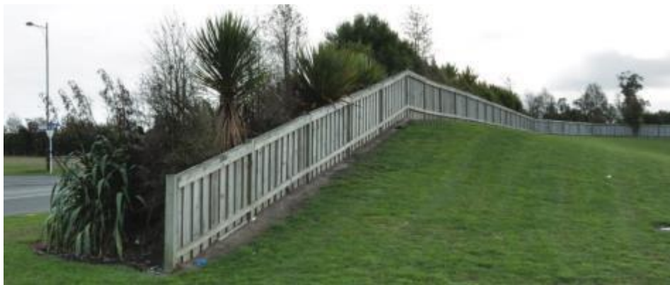
Figure 67: A low height noise wall (timber fence) on top of an earth mound. [158]
