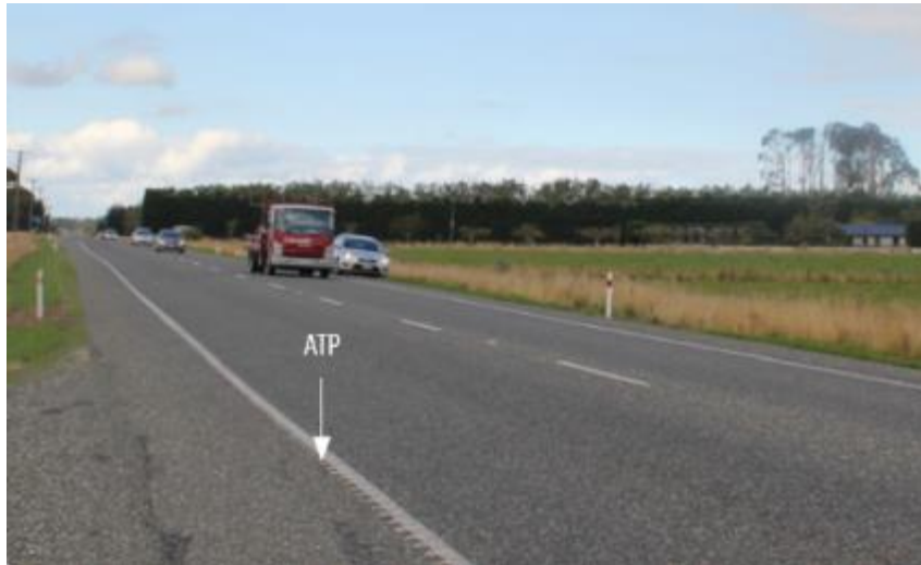
Figure 98: Audio tactile profile (ATP) line marking. (Source: NZ Transport Agency)
