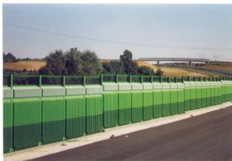
Figure 72: Example of a concrete noise barrier (with transparent panels at the top). A33 Asti-Cuneo, Magliano Alpi, Italy. (Source: G. Magaro' ANAS SpA)
