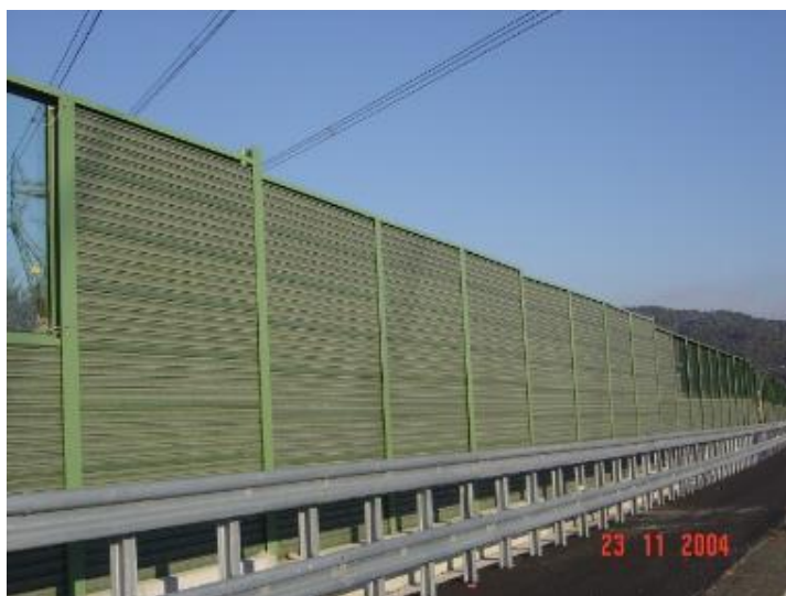
Figure 74: Example of a composite noise barrier. A10 Autostrada dei Fiori, Savona, Italy.
