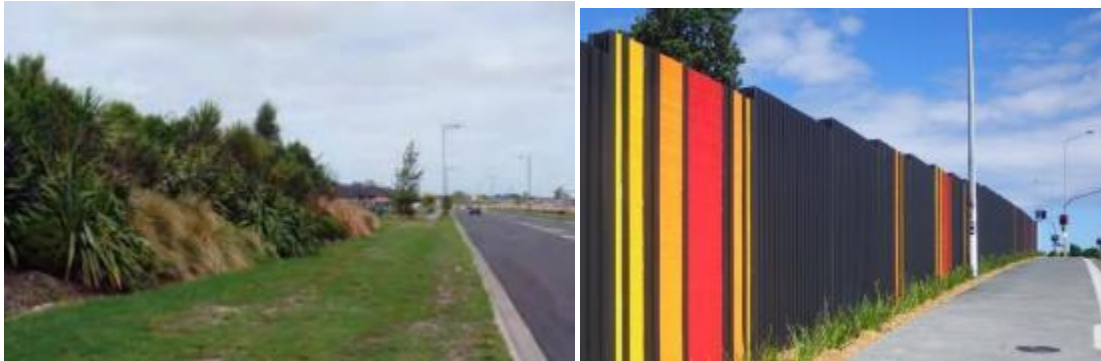
Figure 66: Two types of noise barrier – a planted earth mound (left) and a noise wall (right). [158]
