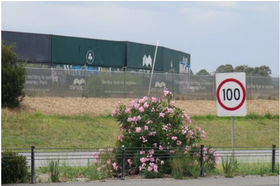
Figure 95: Temporary shipping container noise wall, Monash Freeway, Mulgrave, Australia (Source: J.McIntosh, Department of Transport, Victoria, Australia).
