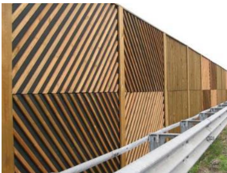
Figure 70: Example of a timber noise barriers A22 Autostrada del Brennero, Rovereto, Italy. (Source: G. Magaro' ANAS SpA)
