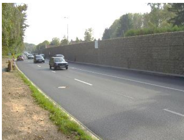
Figure 75: Gabion noise barrier, Westliche Ringstrasse, Ingolstadt, Germany, 2005. (Source: Müller-BBM)
