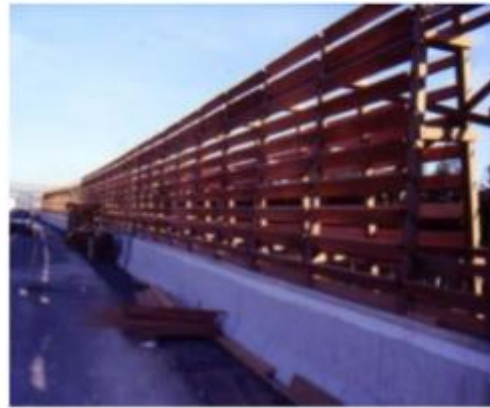
Figure 83: Bio barrier with wooden structure. [165]
