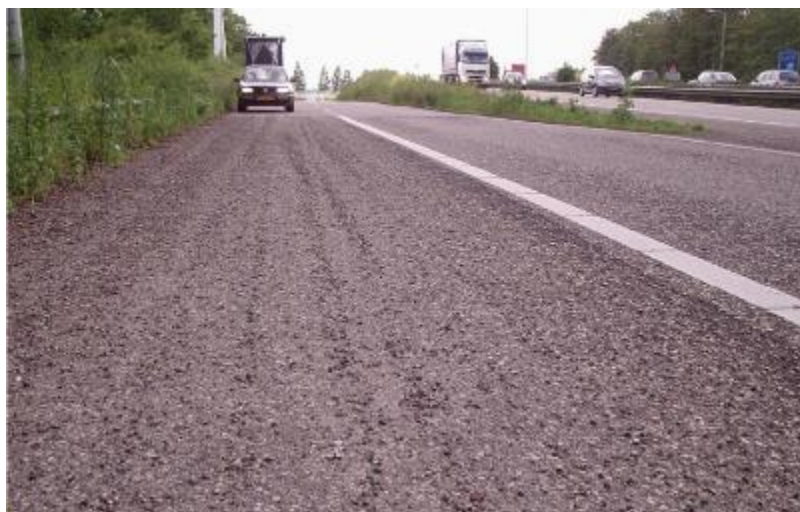
Figure 96: Example of severe ravelling. (Source: Rijkswaterstaat, Netherlands)
