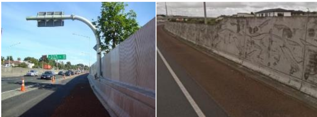
Figure 68: A combined noise and safety barrier (left) and a fully integrated noise and safety barrier (right) (Source: R Hannaby, NZ Transport Agency)
