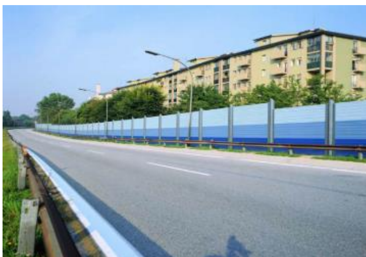
Figure 71: Example of metal noise barriers. Source: A57 Tangenziale di Mestre, Villabona, Italy. (Source: G. Magaro' ANAS SpA).
