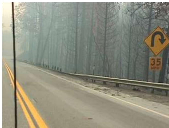
Figure 2.15: Burnt guardrail.
