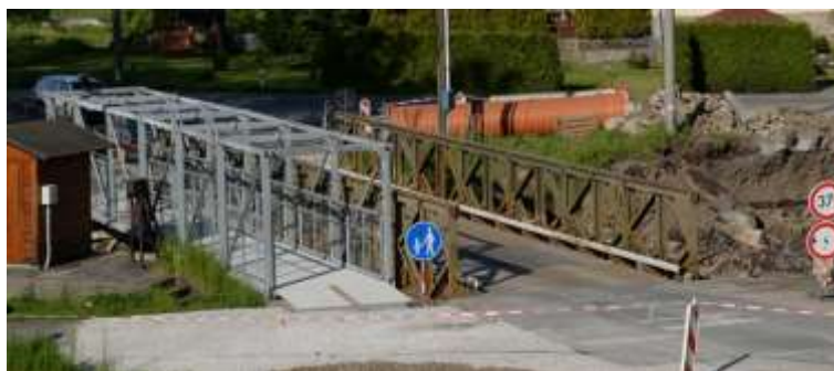
Figure 5.10: Temporary footbridge with span 18.0 m next to the temporary bridge 'MS' (Kozlovice, 2014).
