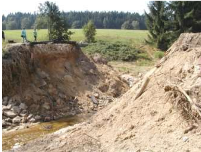
Figure 5.8: Destruction of the bridge structure during the flood of 2002 in the Czech Republic.
