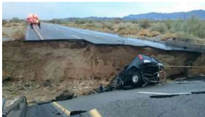
Figure 2.17: Texas Wash Bridge washed out.
