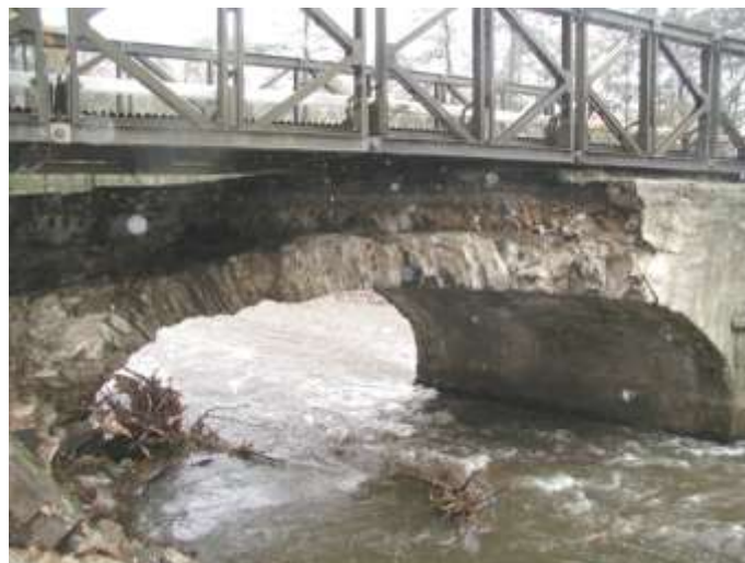
Figure 5.7: Damage to the supporting structure of the bridge due to floods 2002 in the Czech Republic.
