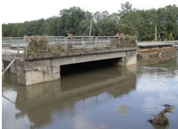
Figure 5.9: Destruction of both access roads to the bridge due to floods 2009 in the Czech Republic.
