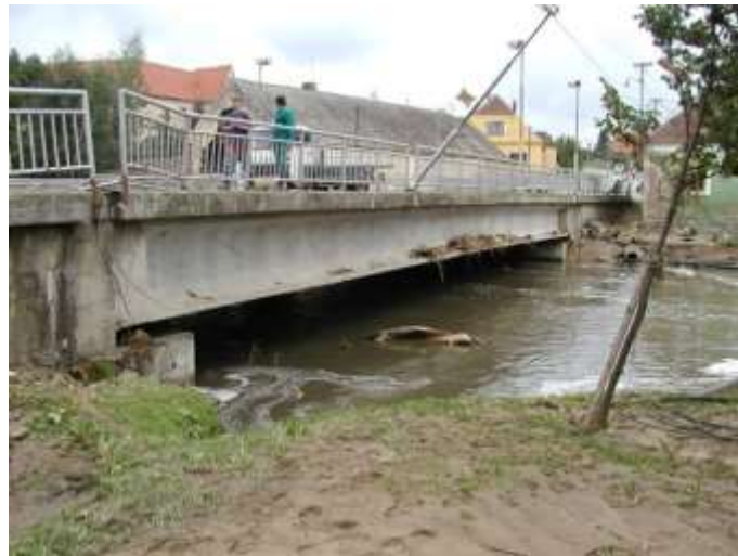
Figure 5.6: Light damage to bridge structure after floods 1997 in the Czech Republic.
