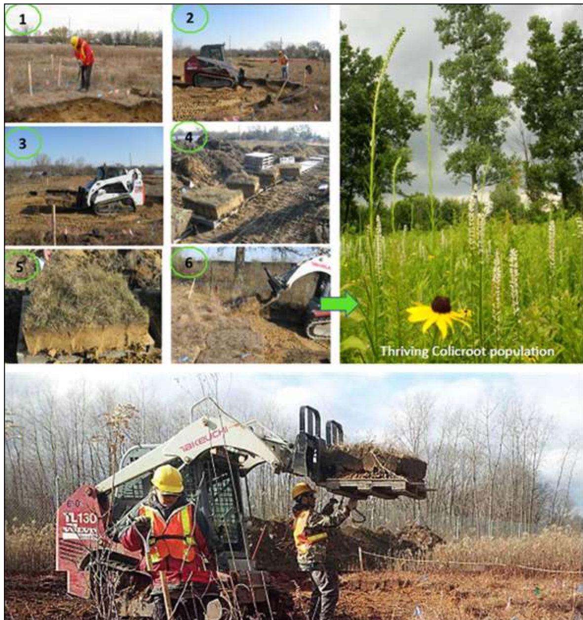
Figure 5: Sod mat transplanting process to protect sensitive prairie grass ecosystem (Ministry of Transportation Ontario, 2016)
