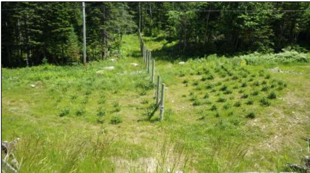
Figure 4. Layout of fence segments at wildlife crossing approaches to promote discovery and use. View a) towards the crossing; b) towards the forest.
