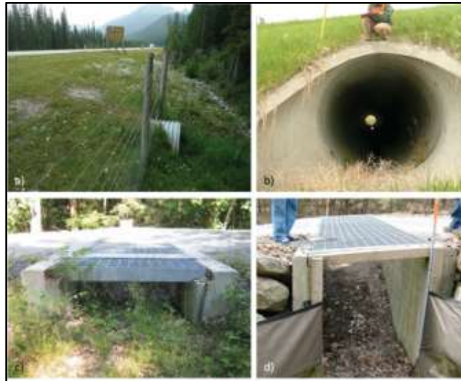
Figure 3: Monitoring underpass structure design for small to medium-sized animals - A vehicle collision with a small or medium wildlife species is less likely to result in human injury or death, but there is high potential for death of the animal. After construction monitoring is essential to ensure wildlife is using the structures put in place (Patriquin et al., 2021; (a) and (b) photo credits: Dr. Tony Clevenger; (c) and (d) photo credits: Kari Gunson).
