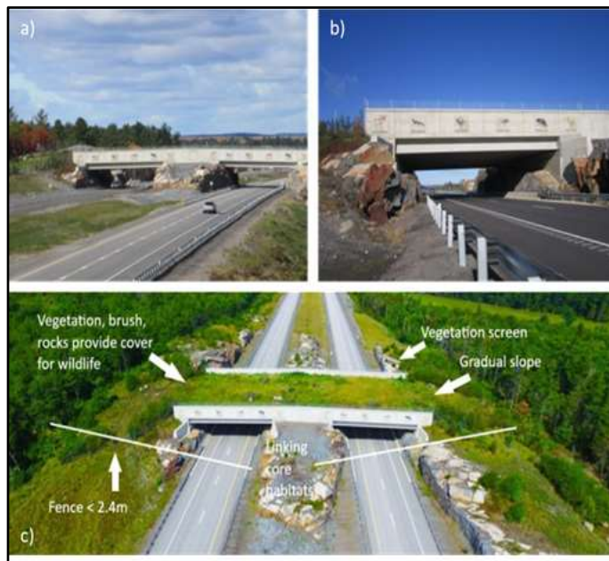
Figure 1: Monitoring overpass structure design – (a); (b); and (c) Highway 69, south of Sudbury, Canada near Highway 637 turn-off to Killarney, Canada. Fencing, roadside vegetation adjacent to crossing structures, and overpass structures requires periodic maintenance. Vehicle and other damage can trigger more significant maintenance costs for fencing and, potentially, overpass structures. This is why monitoring during and after construction is essential (Patriquin et al., 2021; Photo credits: EcoKare International and Ontario Ministry of Transportation).
