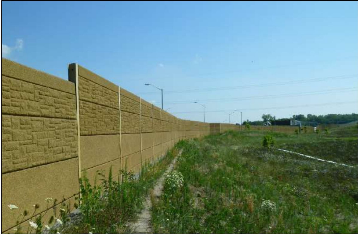
Figure 6: The smooth lower panels of this noise barrier wall prevent Eastern Foxsnakes from accessing the highway (Ministry of Transportation Ontario, 2016)
