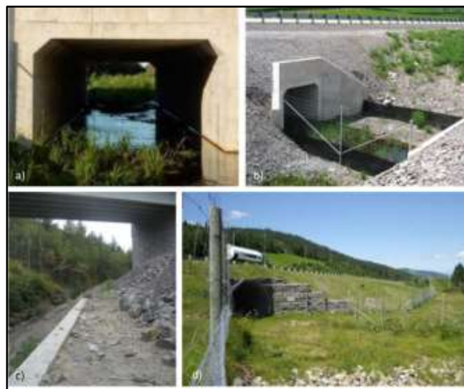
Figure 2: Monitoring underpass structure design – (a) hydrological culvert for aquatic connectivity (Patriquin et al., 2021; photo credit: EcoKare International and Ministry of Transportation, Ontario); (b) fenced aquatic culvert gap (Patriquin et al., 2021; photo credit: EcoKare International and Ministry of Transportation, Ontario); (c) corridor trail below bridge structure (Patriquin et al., 2021; photo credit: EcoKare International and Ministry of Transportation, Ontario); and (d) terrestrial underpass with fencing treatment (Patriquin et al., 2021; photo credit: Martin LaFrance).
